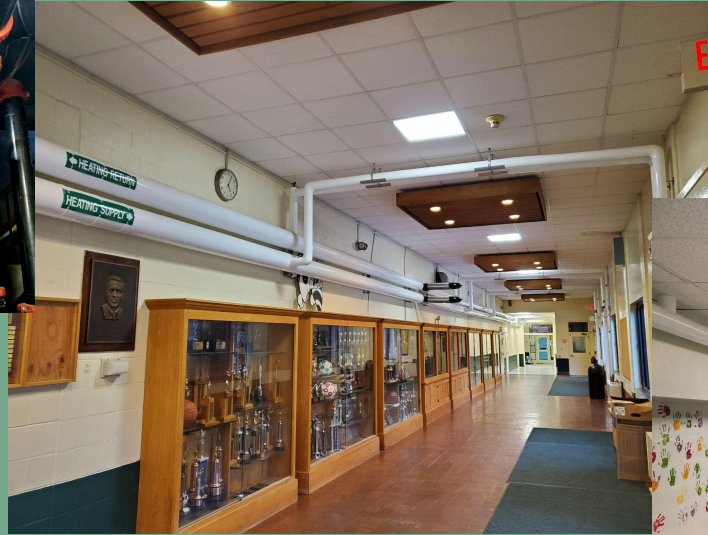
New MS/HS Heating System
