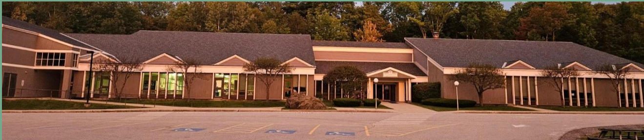
New KES Roof
